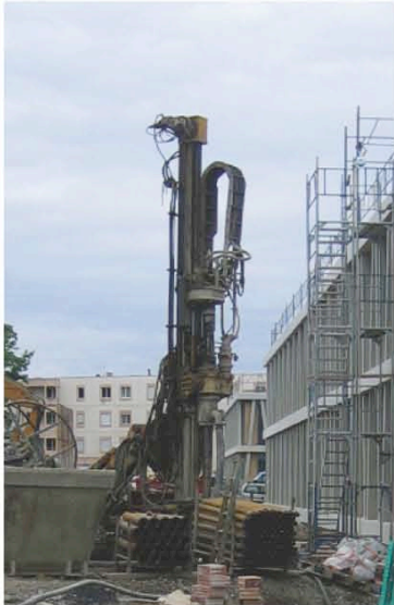
geothermal bore-hole digger
