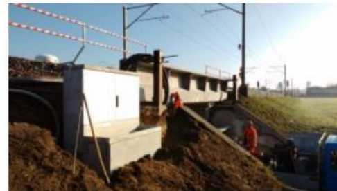
SBB Brücke Sempach – Chatzi (Photo: Interim Report ETH Zürich)
