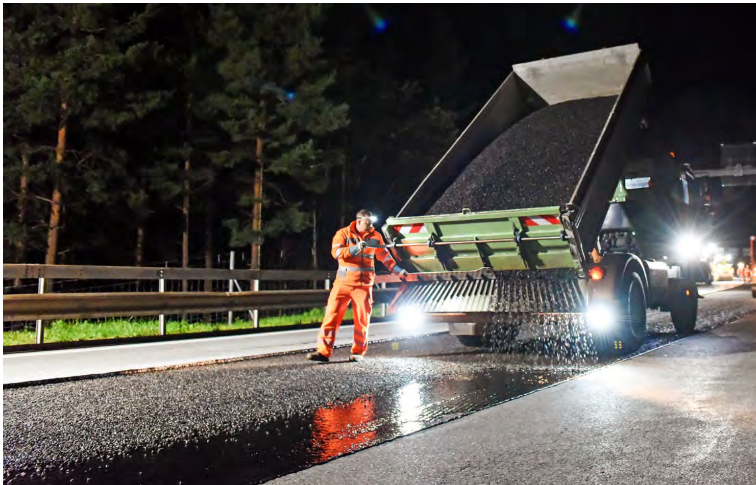
Applikation der SAMI (Stress Absorbing Membrane Interlayer)
