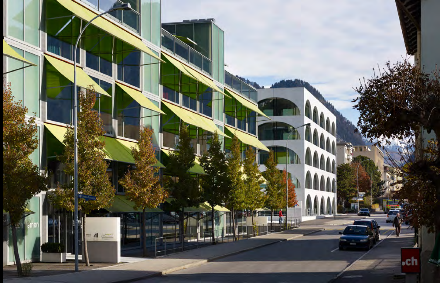
ÖKK office building, Landquart
