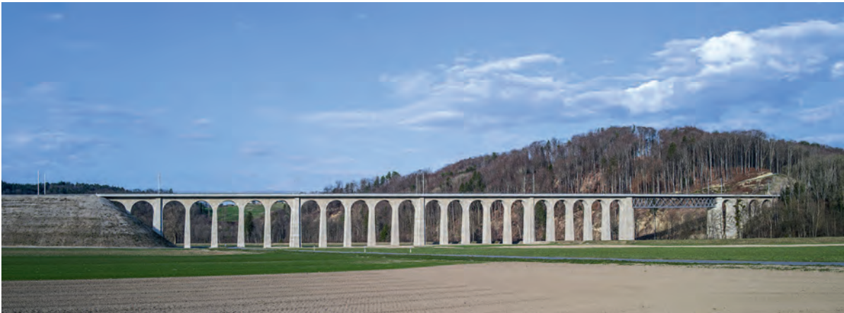
Fig. 7 Vollendeter Doppelspurausbau. Completed double track expansion.
