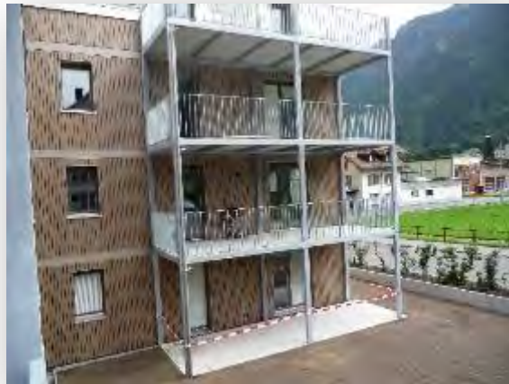
Balkonplatten MFH Linthal
